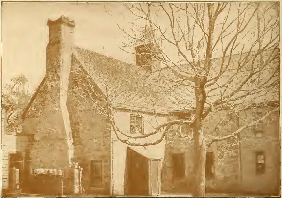
REAR OF SPENCER-PIERCE HOUSE (1651) NEWBURY, MASSACHUSETTS
